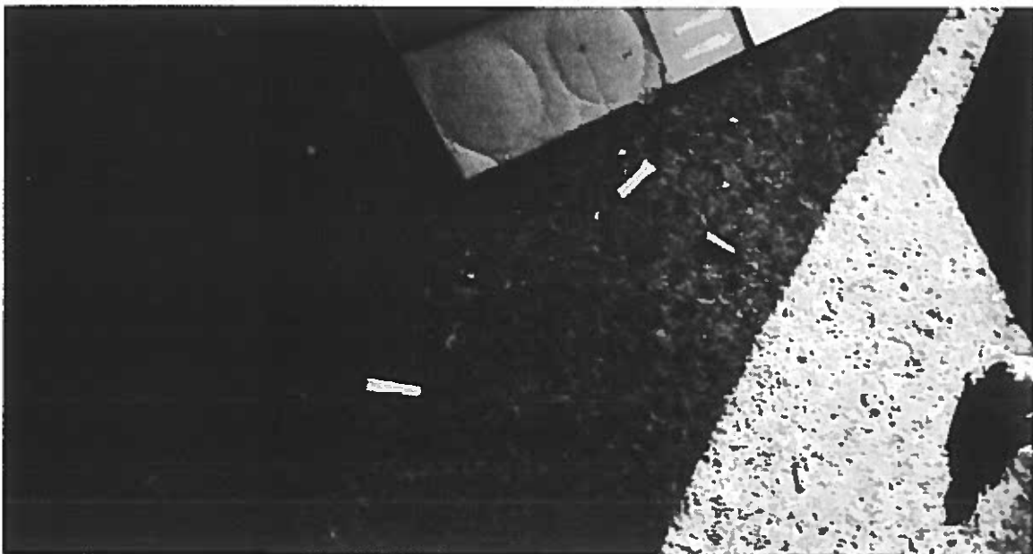
16. The floor of the basement showing discarded cigarettes near to the pile of cardboard boxes shown in image 14.
